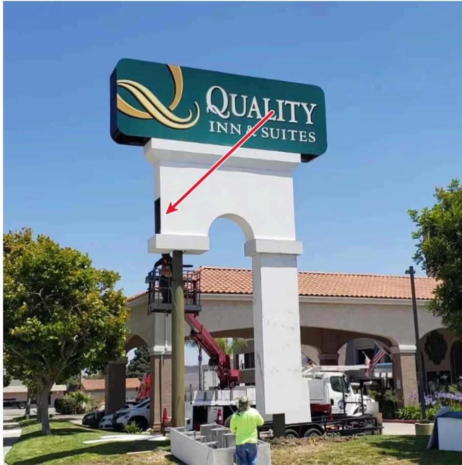
1. Pylon installation · Quality Inn pylon and pole cover. Actual Genius project photo; sample report.
